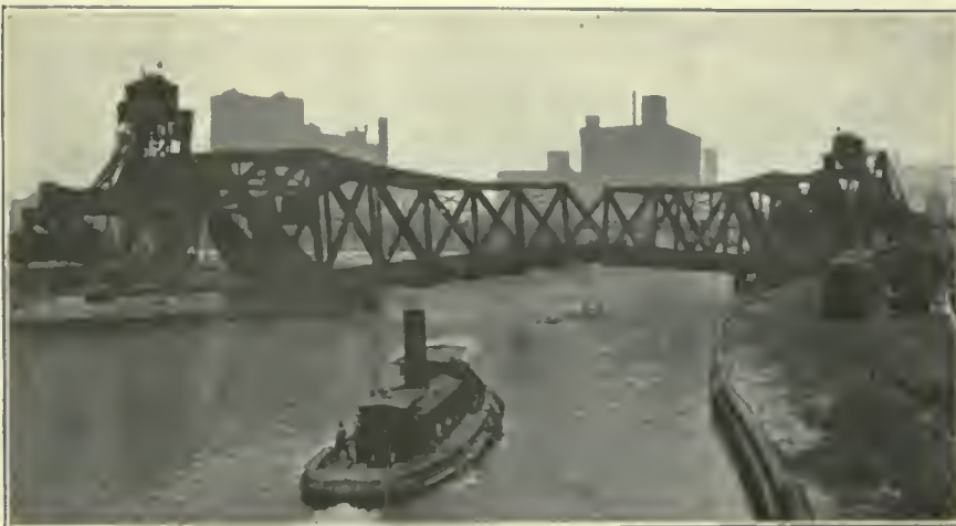
FIG. 265. BRIDGES. Rolling lift bridge of the Baltimore & Ohio Chicago Terminal Railroad over the Chicago River at Taylor Street.
